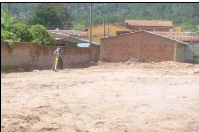
The new building site.
