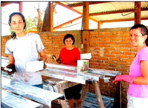
Painting steel "canaletas"
